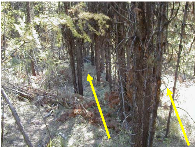
Figure 3.2.3.2.3: Evidence of residual compaction. Note ~ 20 year-old, trees growing primarily in road centerline where there is less compaction. Arrows indicate wheel tracks.
